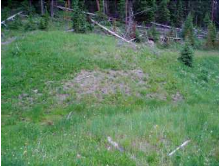
Photo 6. The East Fork of Cache Creek Road was decommissioned in 2002. The culverts were removed, slopes laid back, and the area seeded. The site is completely recovered and the road tread does not have any rill erosion evident.
