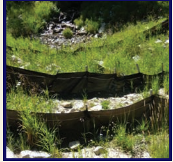
Top A poorly maintained sediment fence (top) allows runoff, while a well designed and maintained fence (bottom) keeps streams clean Below Left Extending the natural vegetative buffer next to the water minimizes nutrient and sediment runoff Bottom Community water quality monitoring
