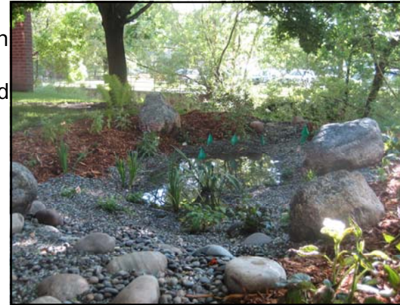
Before (above) and after (below) rain garden installation at the Bozeman City Hall. Rain gardens are landscaping tools to improve water quality and increase water filtration to groundwater.
